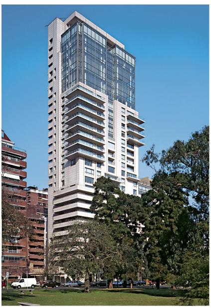
This luxury 33-story residential tower, constructed of steel and concrete and clad in limestone, glass, and aluminum, emerges from the edge of a traditional Japanese garden in an upscale residential neighborhood of Buenos Aires. The building site occupies the leading edge of a residential block that juts out into Parque Tres de Febrero, allowing tenants to look out over parkland on three sides.
